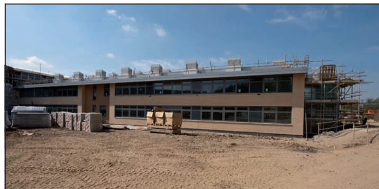
Scaffolding comes down to reveal JCoSS's new building
