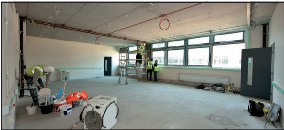
Adding the final touches to one of JCoSS's classrooms
