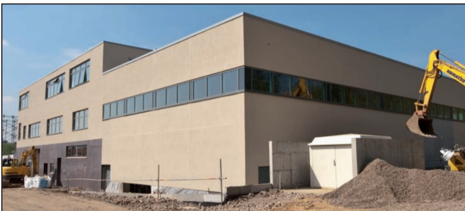
The external work is almost complete
